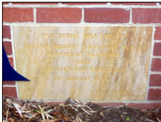
A school foundation stone.
